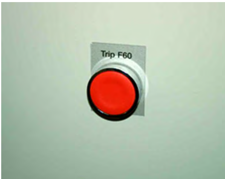
Picture 6 The trip F60 button (pos. 5, Figure 1)
