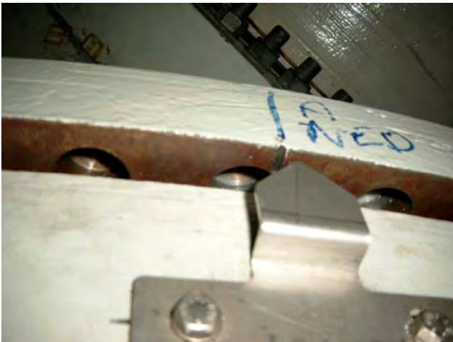
Picture 13 Alignment markings seen from machine foundation side
