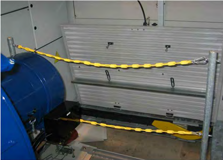
Picture 10 Safety chains must be mounted when the bottom hatch is open (Figure 3)
