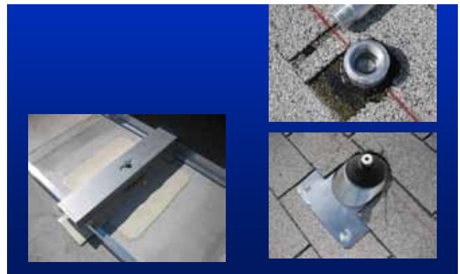
Figure 105. Point attachments connect the array assembly to a building or structure at distributed locations, and are usually the critical design point of the entire mounting system.
